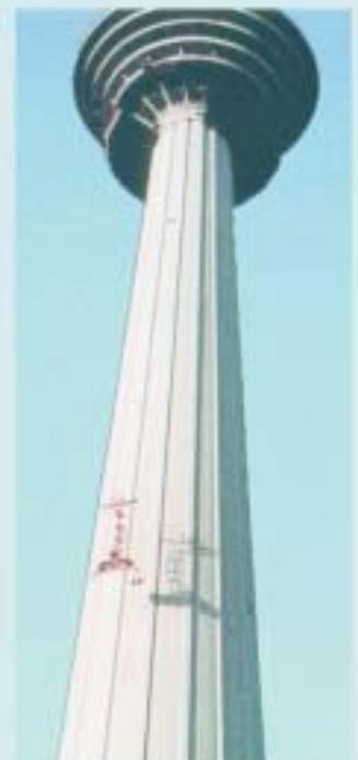
**TIRAK**<sup>®</sup> installed above the load under the upper part of the tower
