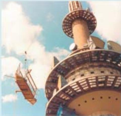
Lifting a component for a **TIRAK**<sup>®</sup> round platform using a return pulley block system.
