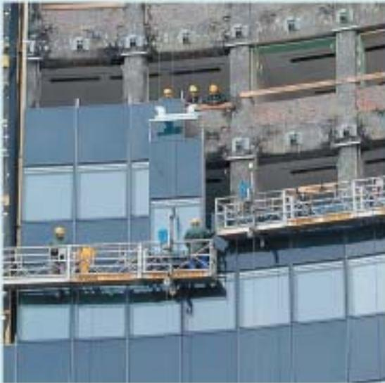
Facade assembly with lifting work platforms. Facade units are moved to the required position in the same way, using **TIRAK®** hoists.
