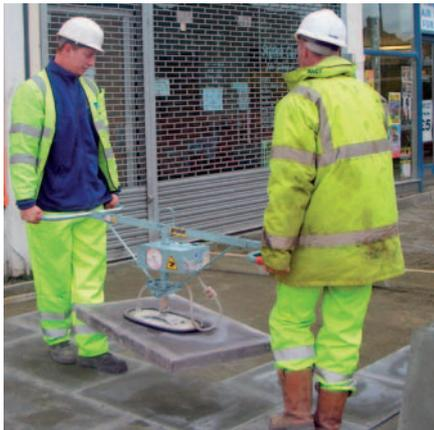
Flexible and powerful hand operated laying device for dense products, such as granite or high quality concrete elements.
